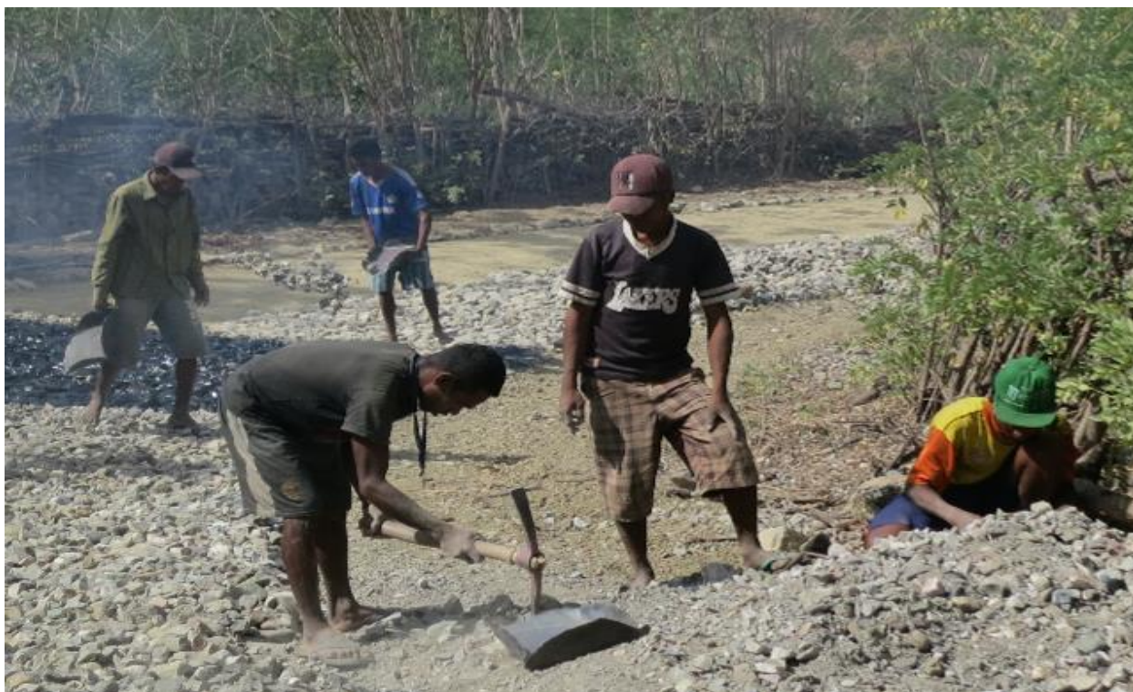
Men repair a local road using stones previously prepared by women
